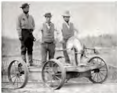
Crank Handcar of Pre-1880 Style; Proved to be Dangerous to Workers
